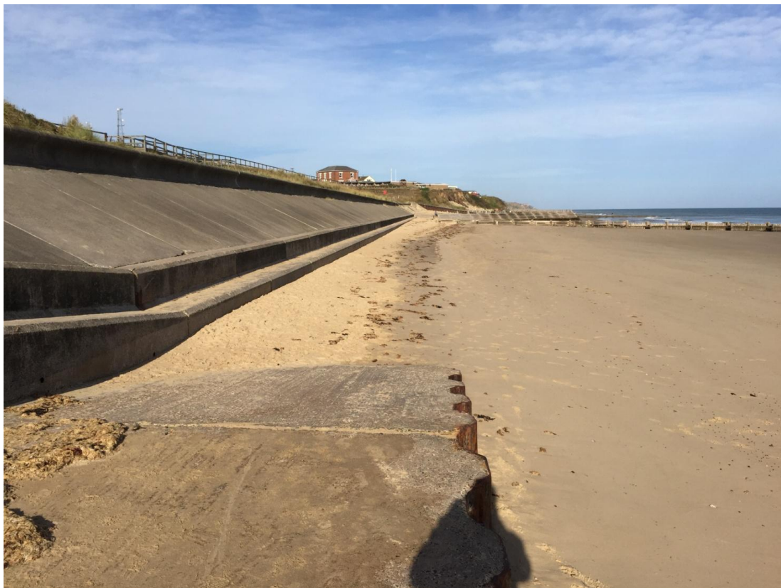
Figure 18. View W-N-W along the sea defence wall showing steel sheet piles at the toe. A timber groyne can be seen projecting into the sea in the distance.
