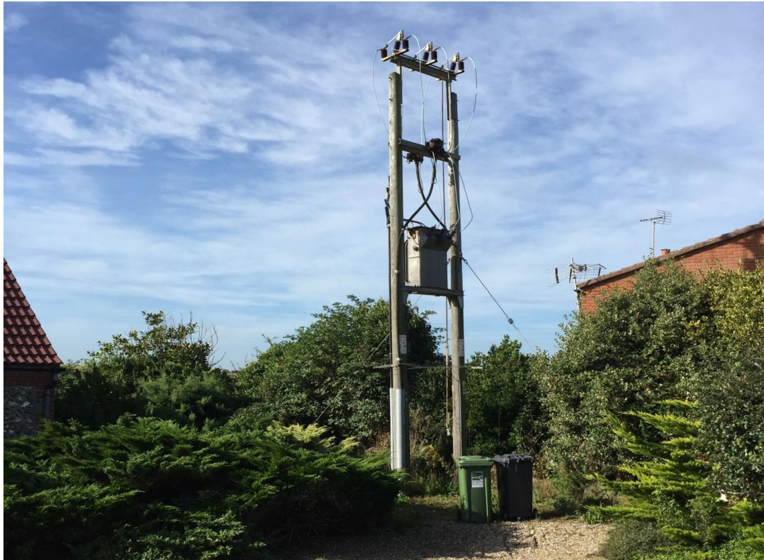
Figure 13. Transformer for underground cables located on the opposite side of the B1159 Coast Road from the site. The transformer can also be seen in Figure 10.
