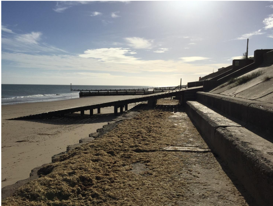
Figure 17. Timber beach access ramp at Bacton Gap.
